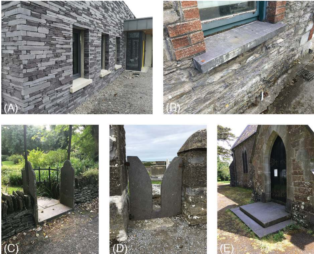
Fig. 10—Uses of Valentia Slate: (A) Modern construction stone; (B) Window sill; (C) Gate piers, Knightstown; (D) Wall Stile, Ardferit; (E) Steps and roofing slates, St John's Church, Knightstown.
