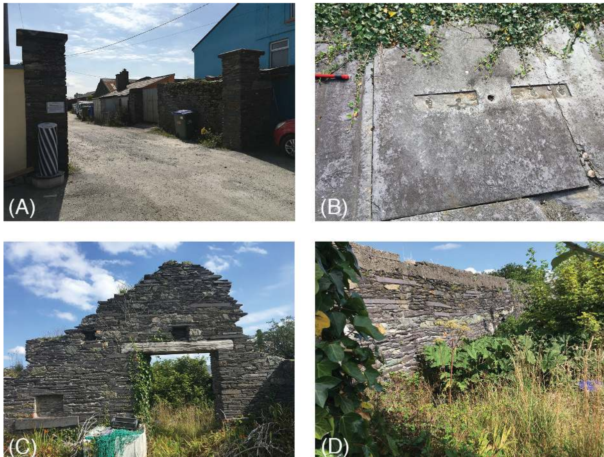
Fig. 7—Valentia Slate Yard. (A) Entrance; (B) Slab floor of demolished engine room with carved recesses for machinery; (C) The First Message building used for hand cutting slate or as a store; (D) Interior of the First Message building showing construction style in Valentia Slate.
