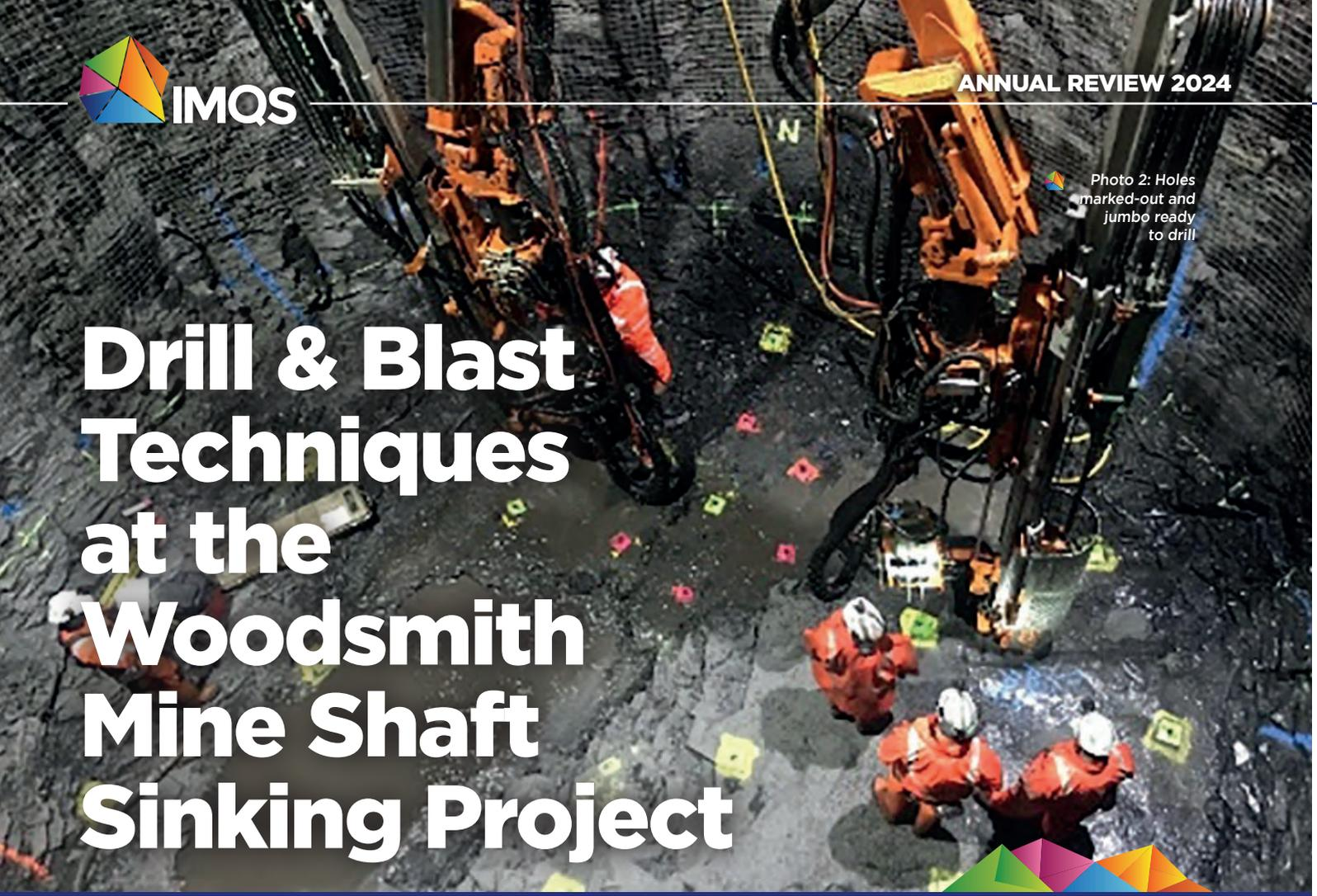
Photo 2: Holes marked-out and jumbo ready to drill
