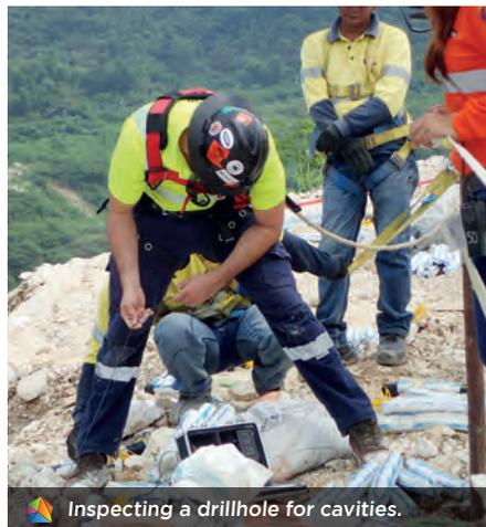
Inspecting a drillhole for cavities.
