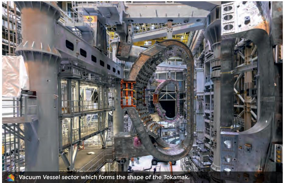
Vacuum Vessel sector which forms the shape of the Tokamak.
