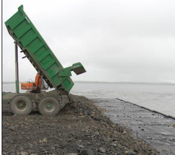
Placement of Rock Cap
