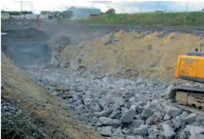
Fig. 17 – Work to seal the portal section on top of the decline plug on the decline.
