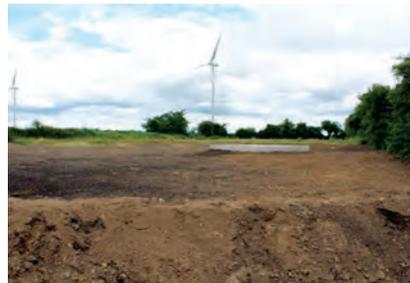
Fig. 13 – Vent Raise 9 – Backfilled and rehabilitated.
