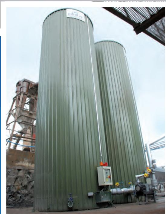
2 x 77m<sup>3</sup> vertical energy efficient bitumen tanks with turbine stirrer
