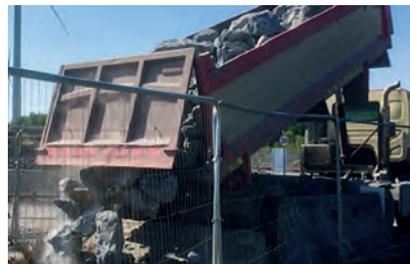
Fig. 11 – Tipping rock into a vent shaft.
