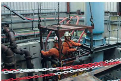
Fig. 9 – Workers access the Fresh Air Shaft to assist with the removal of the Alimak Emergency Exit equipment from the Mine.
