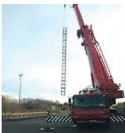
Fig. 10 – Removal of a section of the Alimak from the Fresh Air Shaft.
