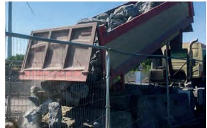
Fig. 11 – Tipping rock into a vent shaft.
