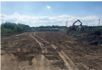
Fig. 18 – The completed decline / portal plug – covered over with overburden.
