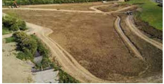
Fig 3. Both ICW cells completed and topsoil in place during initial planting. Note the channel along the Southwest boundary, directing through-flow from Cell 1 to Cell 2 (May 2017).
