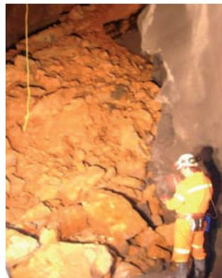
**Face collapse, weathered sands/clays, with no cohesion and no strength**
