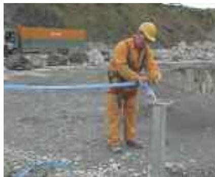
Two tensionable fibre straps are connected between poles up to 20 metres apart.
